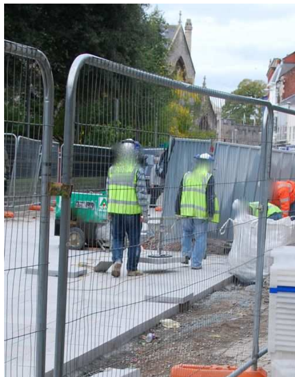
(Photo: Richard Neale Skanska project, Cardiff, Wales, UK)
