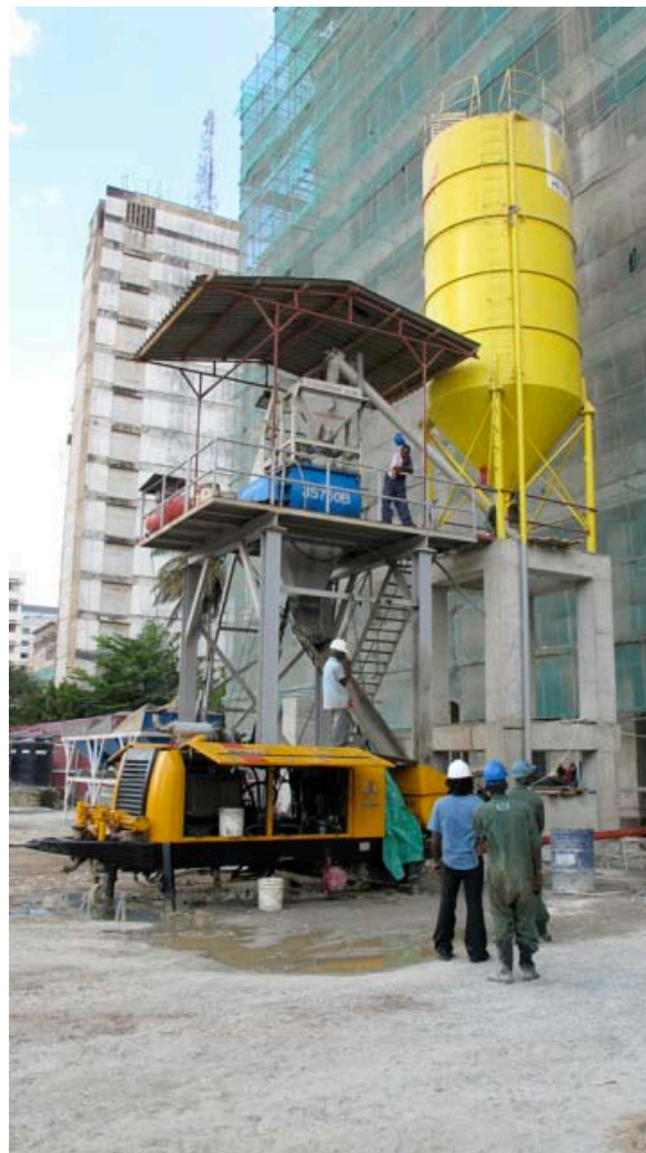
(Photo: Richard Neale. Project in Dar es Salaam)
